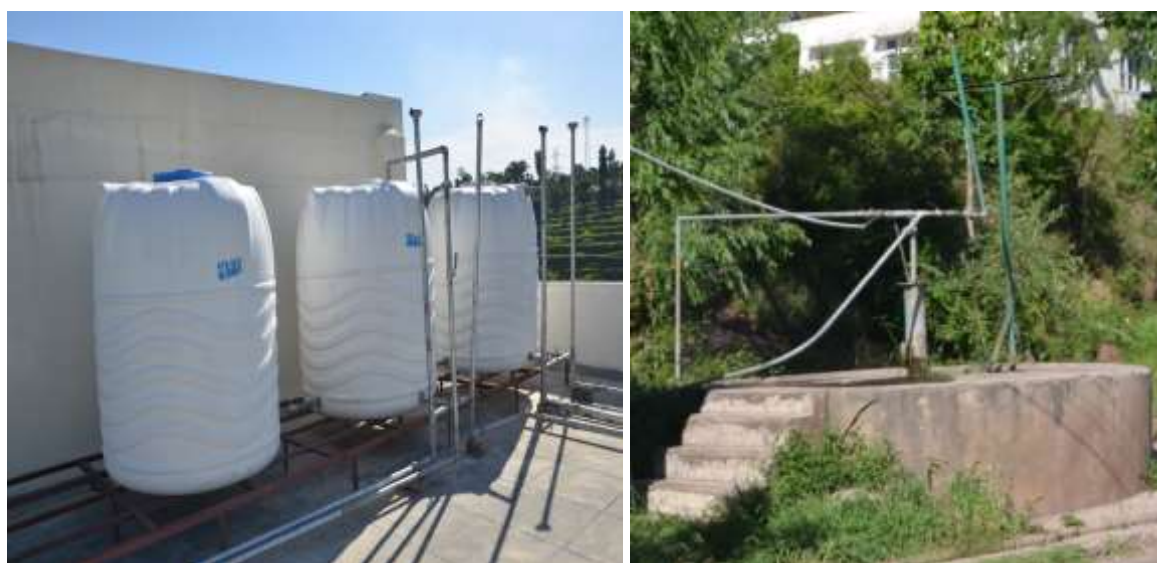
Plate 4. Water tanks in the University and Borewell near Sabrang Square
