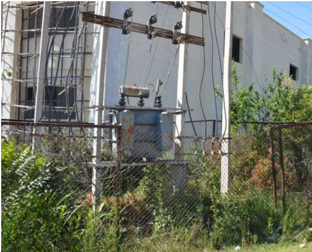
Plate 2. Hydroelectric power transformer installed near Lead Garden/New Library building
