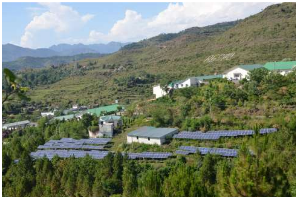
Plate 1. Solar Power Plant, BGSBU
