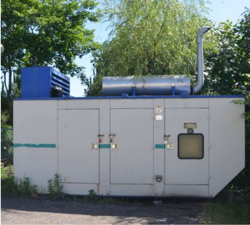
Plate 3. A diesel generator installed near School of Biosciences and Biotechnology
